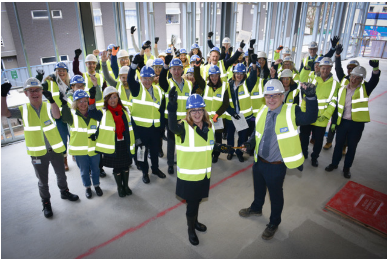
Critical Care refurbishment is underway
