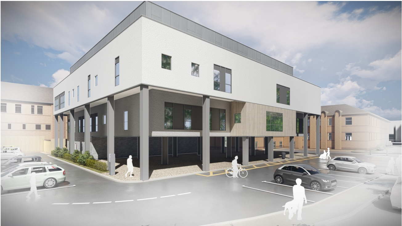
New Ophthalmology centre being built
